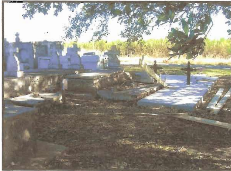
Above: New concrete pads in the cemetery
